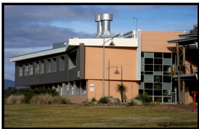
A phase change wax product has been embedded into the walls and floor of this office building. The material absorbs and later releases heat to modulate changes in temperature.
