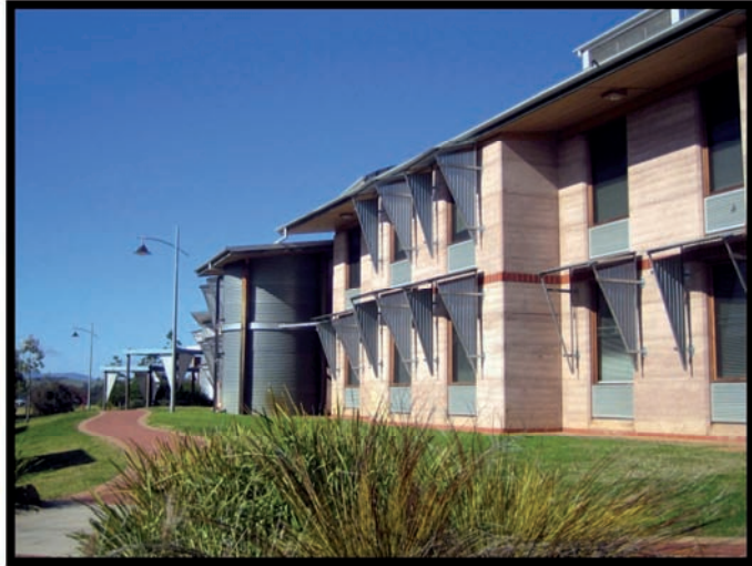
This rammed earth office building has walls constructed by compressing a wet mix of natural materials into a frame. This delivers walls that are durable with high thermal mass.
