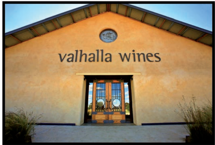
Valhalla Winery, Wahgunyah, was constructed in 2007 from jumbo straw bales. After the bales were laid, 3 coats of lime render mix were pumped onto the surface to protect the bales. The design includes many passive design and sustainability features.
