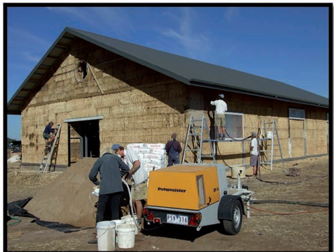
Valhalla Winery, Wahgunyah, was constructed in 2007 from jumbo straw bales. After the bales were laid, 3 coats of lime render mix were pumped onto the surface to protect the bales. The design includes many passive design and sustainability features.
