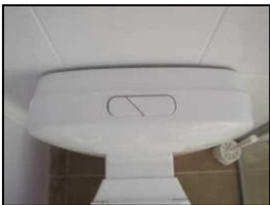
Figures 12 & 13: Dual flush toilet cisterns can be installed as a new unit or retrofitted separately to the existing toilet assembly. Low flow shower head.
