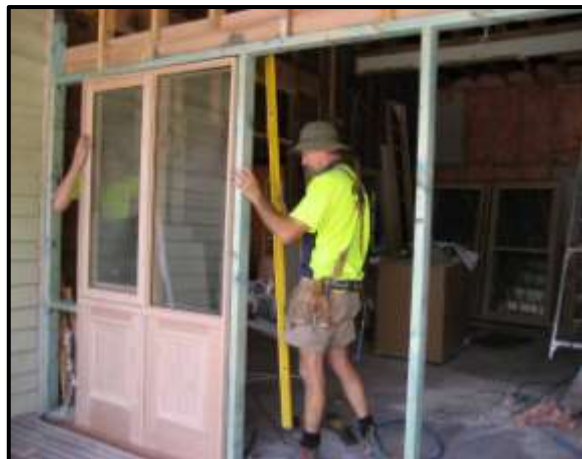
Figures 2. Double glazed windows and French doors being installed.
