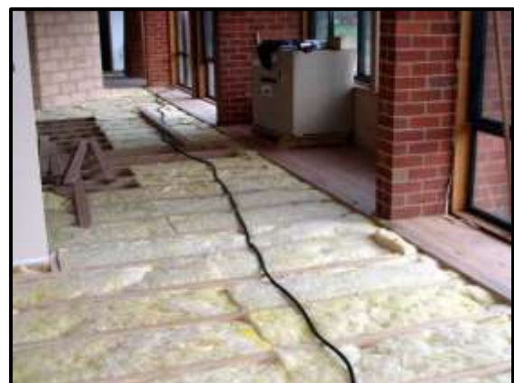
Figure 8: Floor insulation can minimise heat transfer through wooden floor boards.
