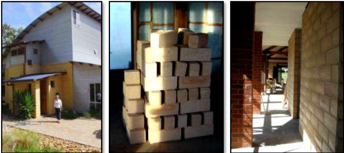
Figure 28-30 Left-right: Timbercrete and metal clad home, Timbercrete blocks, and a reverse veneer Timbercrete build with additional clay brick structures to enhance internal thermal mass.
