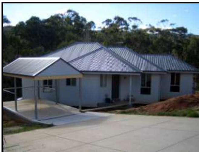
Figure 25: An AAC panel home. The panels have been finished with a render to seal the material.
