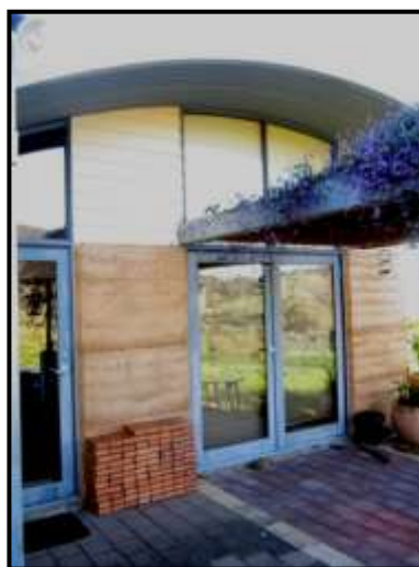
Figure 27: Rammed earth wall
