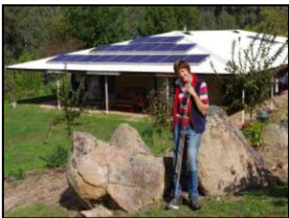
Figure 14: A roof mounted solar PV array that produces half of this homes annual electricity requirements.
