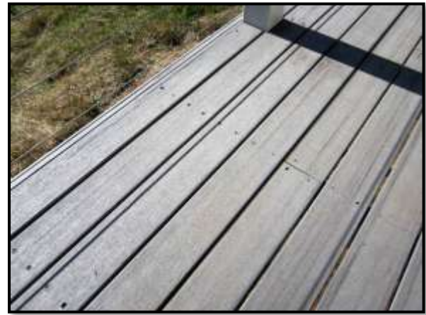
Figures 10: A wood composite product was selected to use in the building of a new deck. The timber look-a-like product is made from recycled timber and plastic and has the look and feel of timber but without the traditional maintenance requirements.
