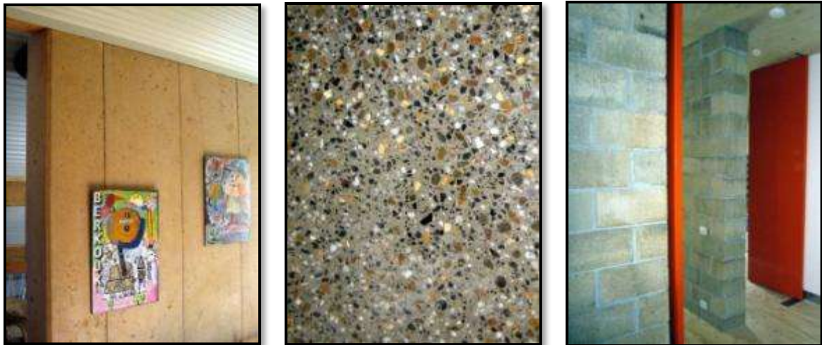
Figures 5-7. Thermal mass used within homes. Left to right. Internal poured earth wall, polished concrete floor, concrete brick walls.
