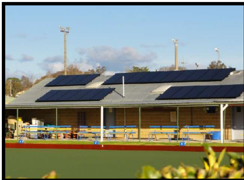
A 4.94 kW solar panel system was installed on the roof of the Kiewa Bowls Club at Coulston Park, Tangambalanga. The saving from the system will be shared by all of the user groups at the complex.
