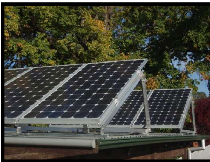
Frames used on a flat roof to correct tilt and orientation.
