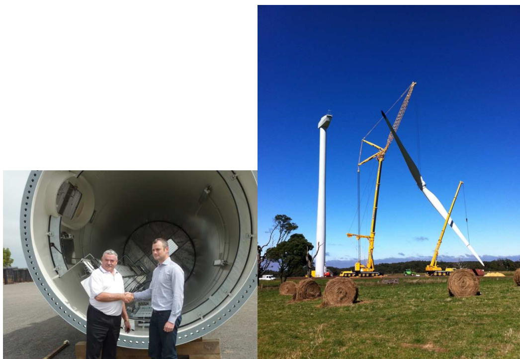
Figure 7. Hepburn community wind project at Leonards Hill near Daylesford....local manufacturing jobs for the turbine stands and raising the first turbine in April 2011 2 .
