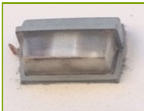
Photo: External mercury vapour lights to be replaced with LED
